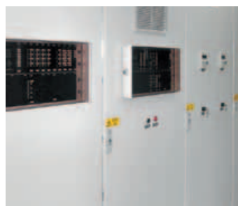
From left to right: Gas burner, heating circuit manifold, switchgear
