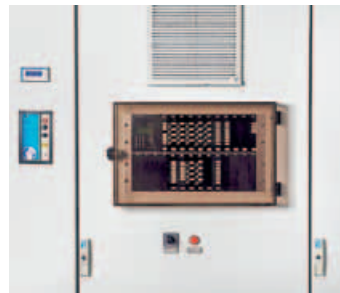
From left to right: Modernised boiler house with new burners, burner fitted with frequency converter, PLC control of the multi-boiler control system
