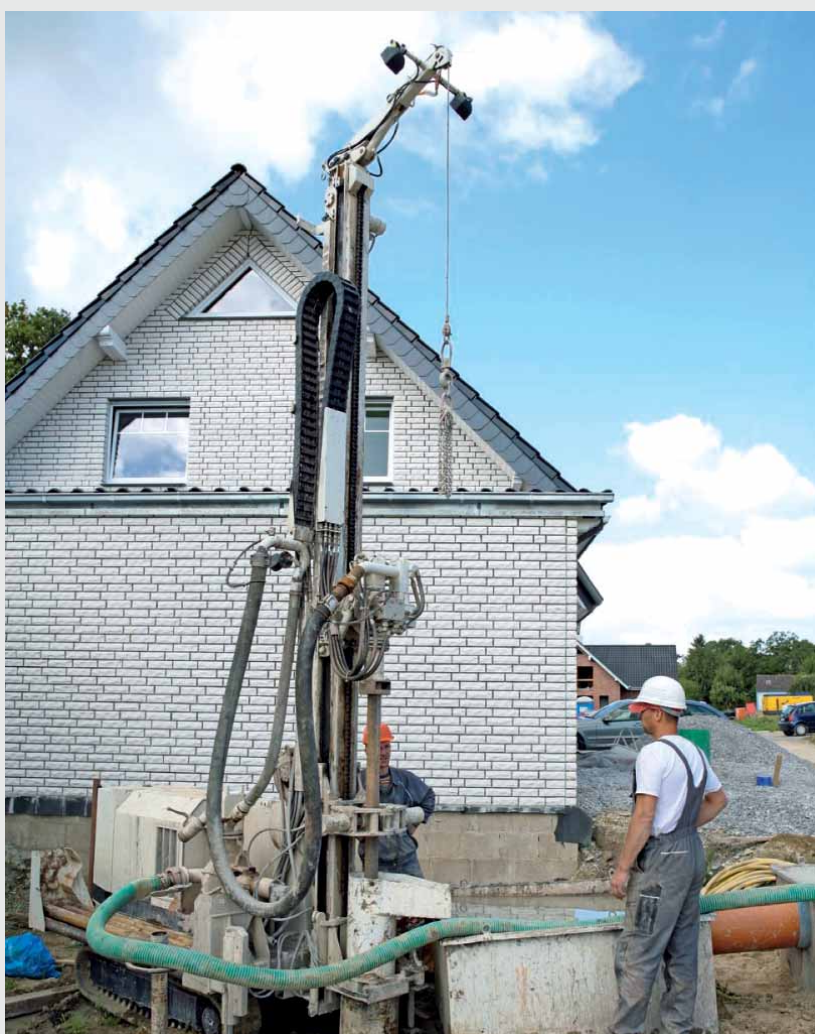
Bore-hole for geothermal heat exchanger
