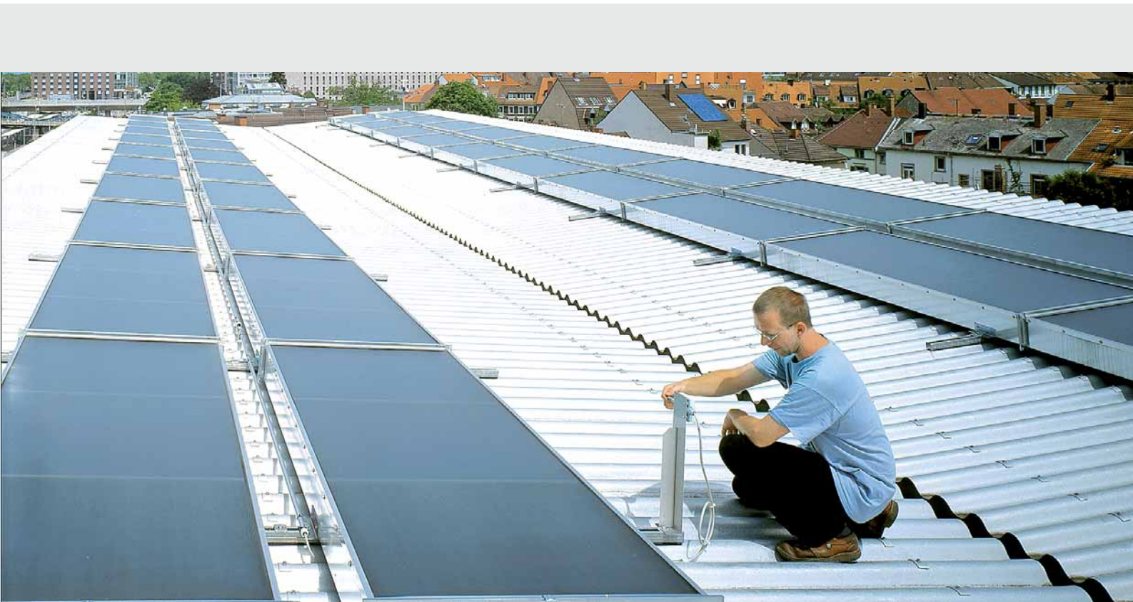
Example of solar cooling
